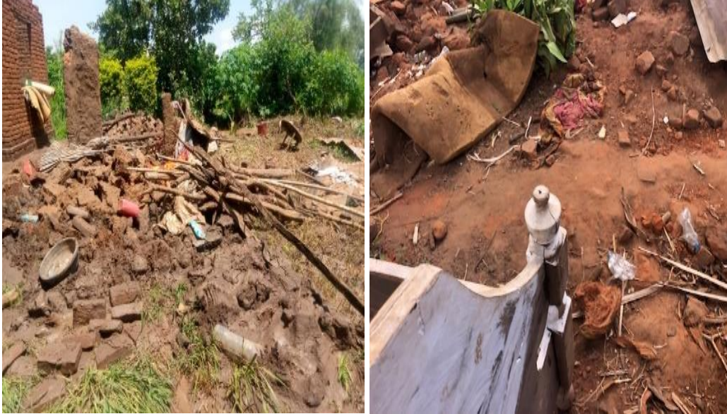
Photos 2 & 3: Houses and Belongings Destroyed by Floods Completely in February 2022
