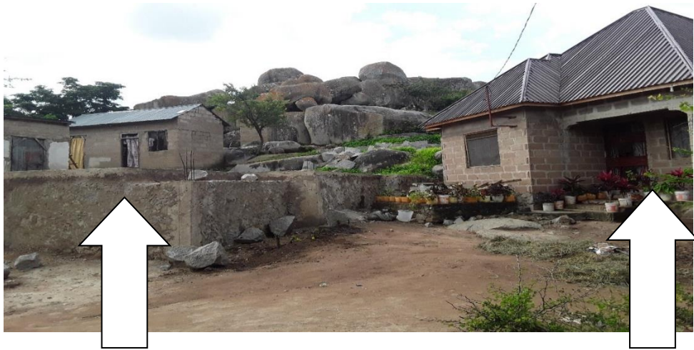
House built before (2016)
